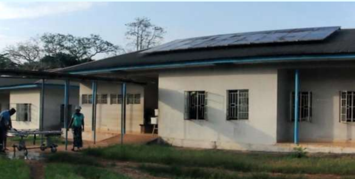
Solar power Community Hospital, Serabu, Sierra Leone, 2017
