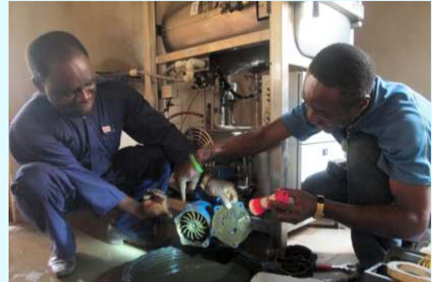
Sterilizer repair, Umuowa Hospital, Nigeria 2013
